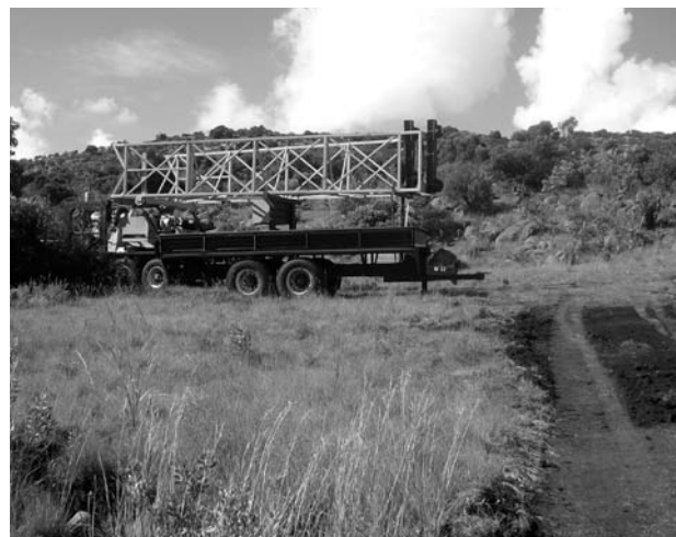
Derrick being deployed on the Southern Cluster.
